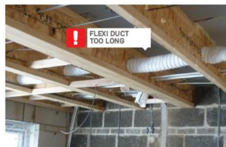
FLEXI DUCT TOO LONG AND NOT SUPPORTED = FANS WILL BE NOISY / INEFFICIENT VENTILATION COMMISSIONING NOT DONE CORRECTLY
